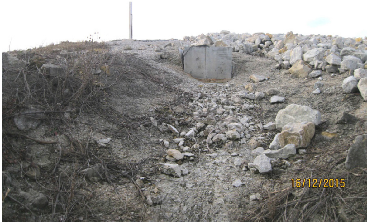
Figure 4-5 Exterior Dike Slope Surface at Discharge Pipe.
