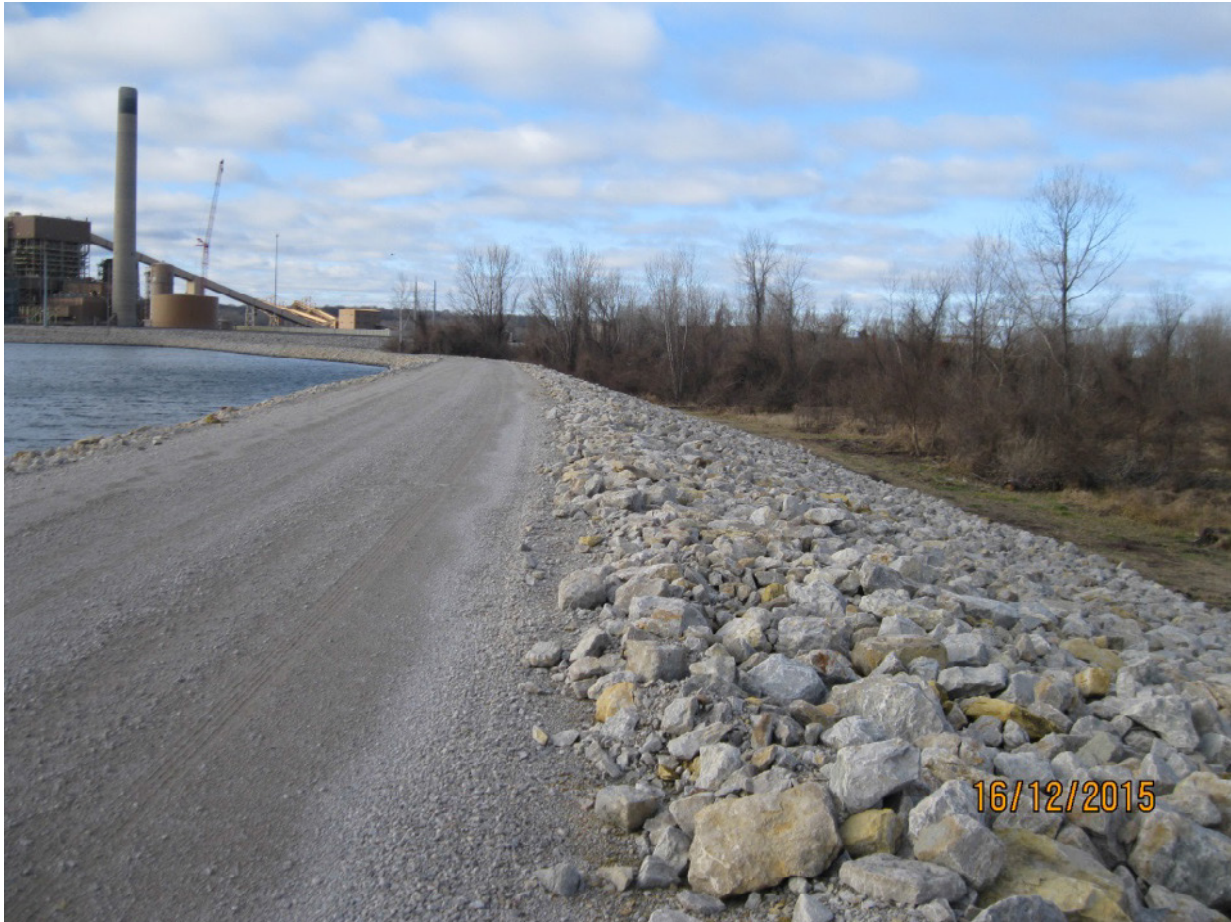
Figure 4-1 Exterior Dike Crest Condition
