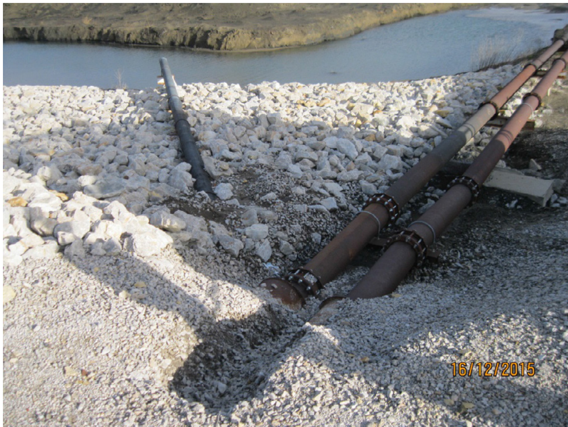
Figure 4-10 Minor Erosion Along Bottom Ash Sluice Pipes
