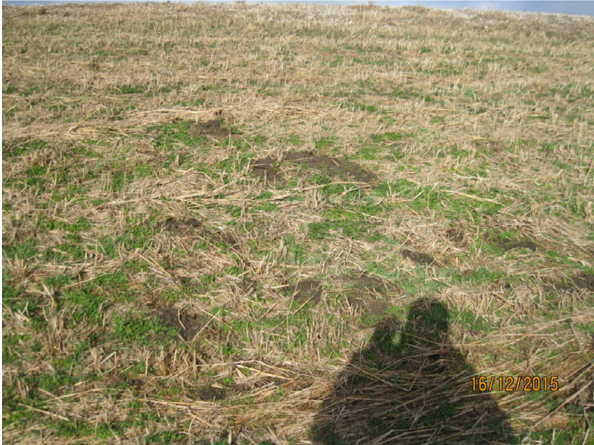
Figure 4-8 Minor Surface Disturbances Along the Southeast Facing Exterior Slope.
