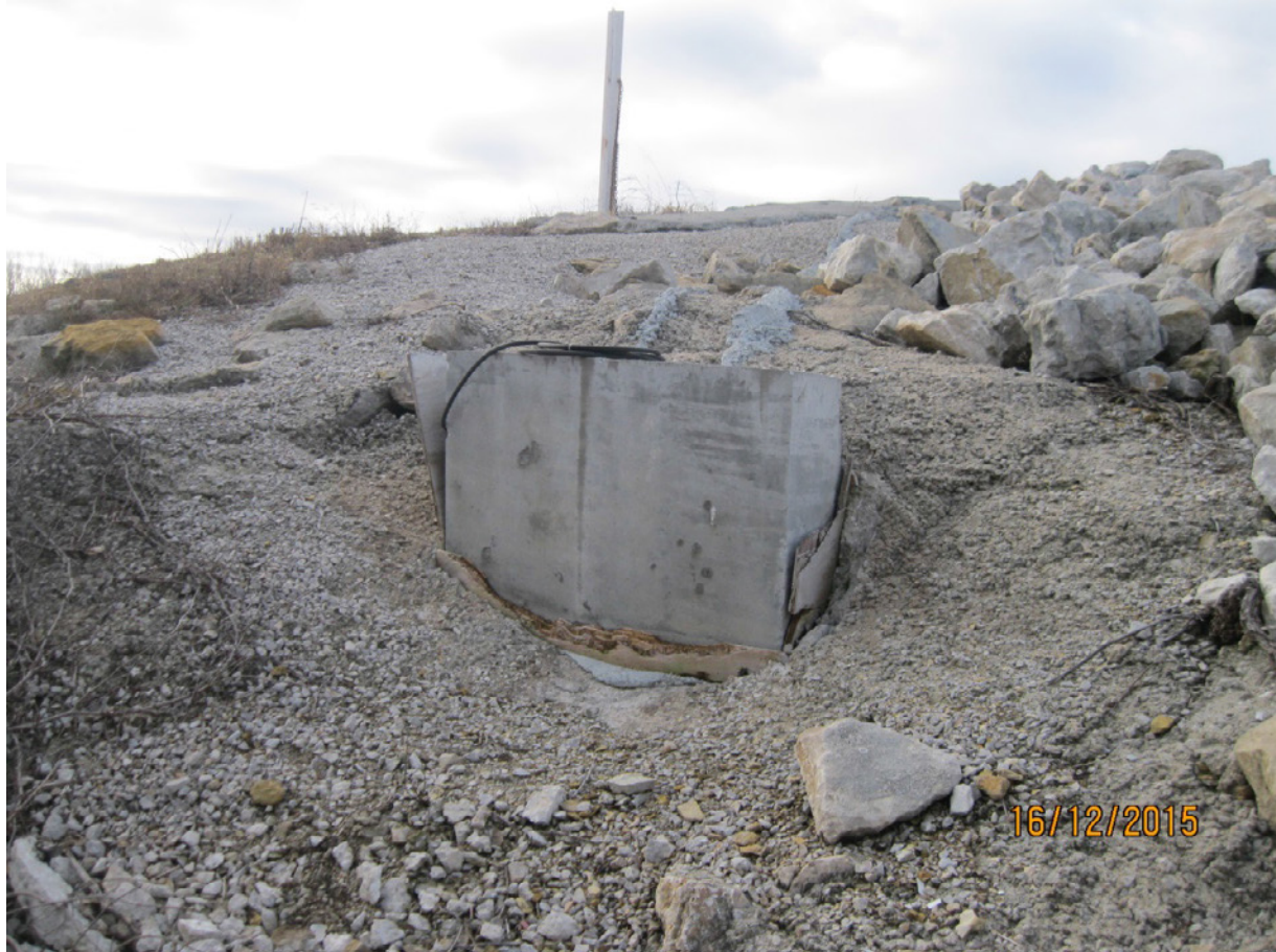
Figure 4-9 Bottom Ash Pond 30 Inch Diameter Discharge Pipe.
