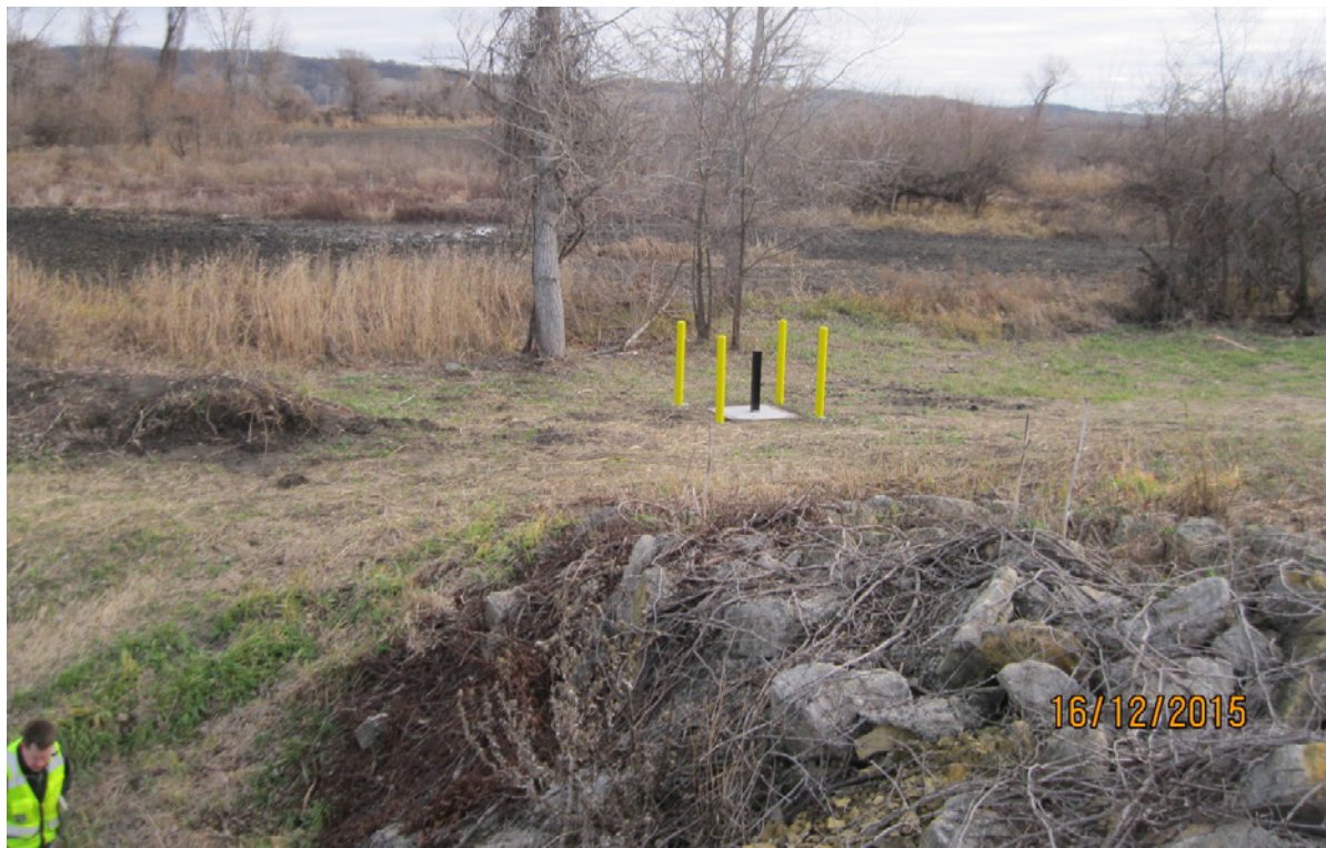
Figure 4-6 Exterior Dike Slope Surface East of the Discharge Pipe.
