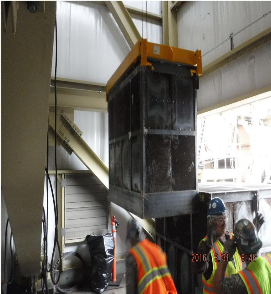
Catalyst facilitates NO<sub>x</sub> removal in the presence of ammonia.
