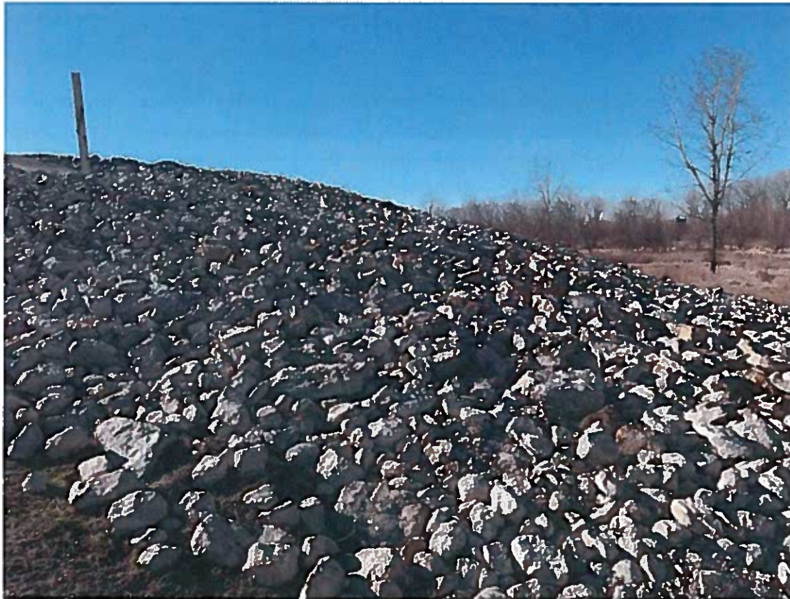
Figure 4-3 Exterior Dike Riprap Placement.
