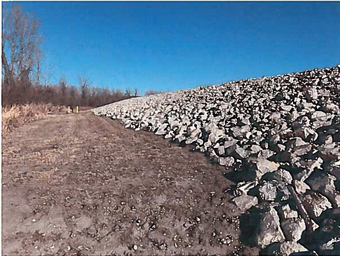
Figure 4-2 Exterior Dike Slope in North Facing Slope of Impoundment
