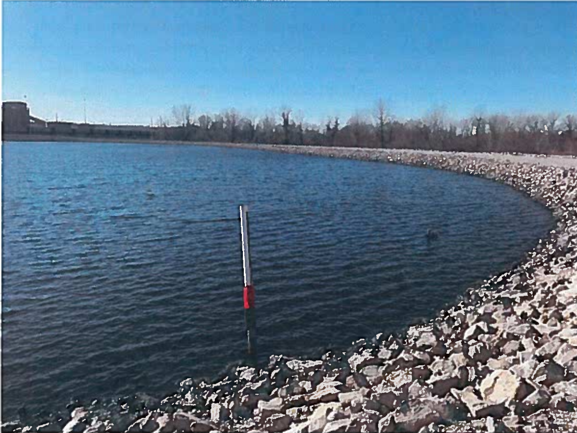
Figure 3-1 Water Level Indicator
