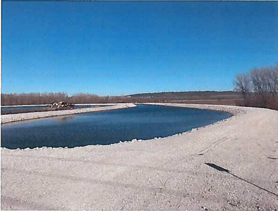
Figure 4-1 Interior Dike Crest Condition
