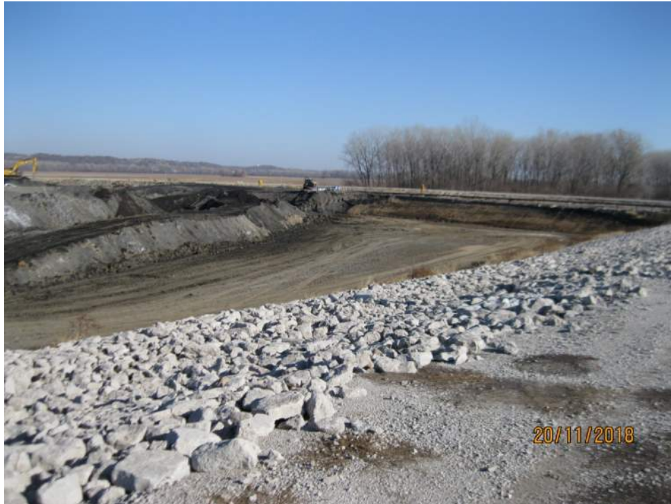
Figure 7 – Shaping of Interior Slopes as Bottom Ash is Removed.
