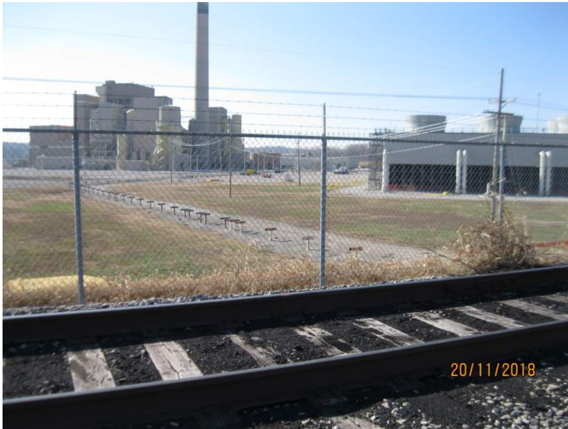
Figure 2 – Remaining Pipe Supports along Sluce Pipe Alignment.
