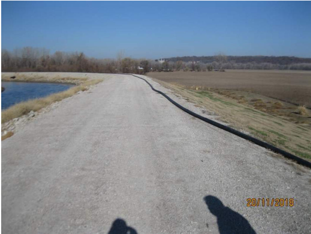
Figure 6 - Clear Water Pond Dike Crest Condition
