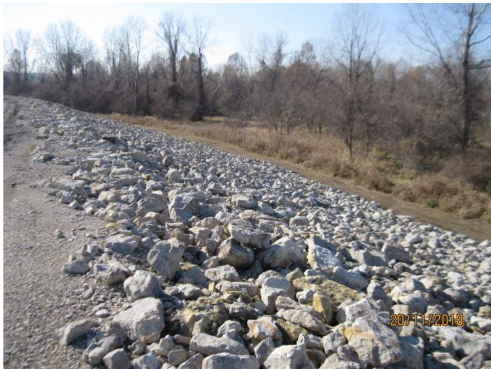
Figure 5 – Rip Rap on Exterior North Dike of Bottom Ash Impoundment
