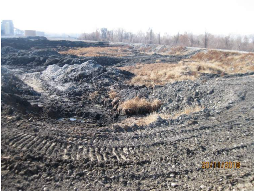
Figure 3 - Dry Condition of Bottom Ash Impoundment
