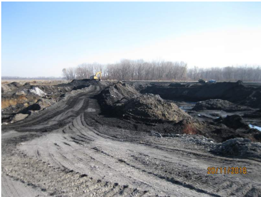
Figure 1 – Dry Bottom Ash Impoundment – Removal by Backhoe and Dump Trucks
