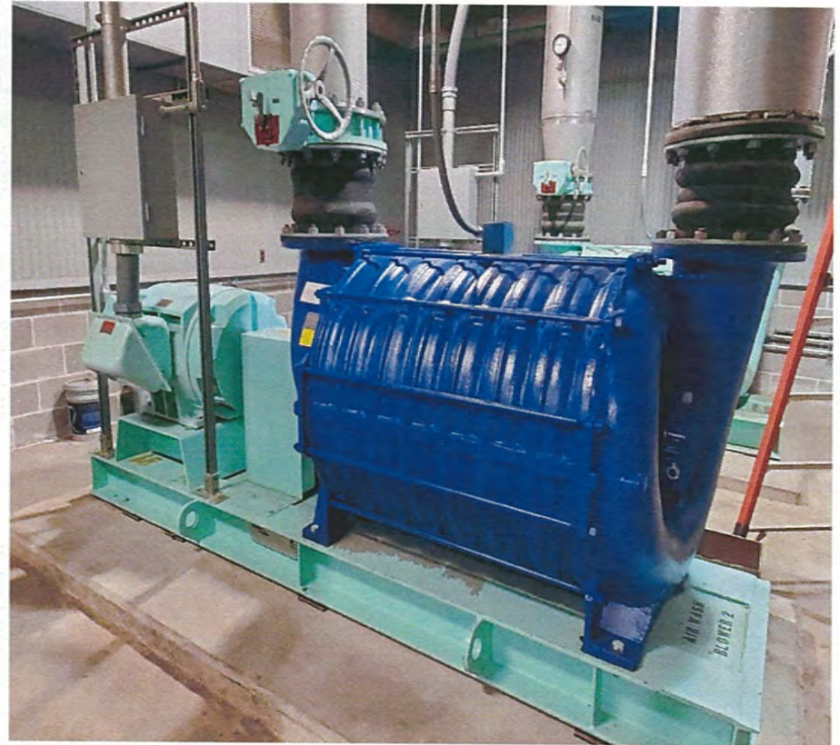
Rebuilt blower unit
