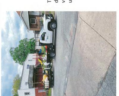
The use of pressurized water to crate a dirt slurry. The equipment can then vacuum the slurry to reveal buried utilities.
