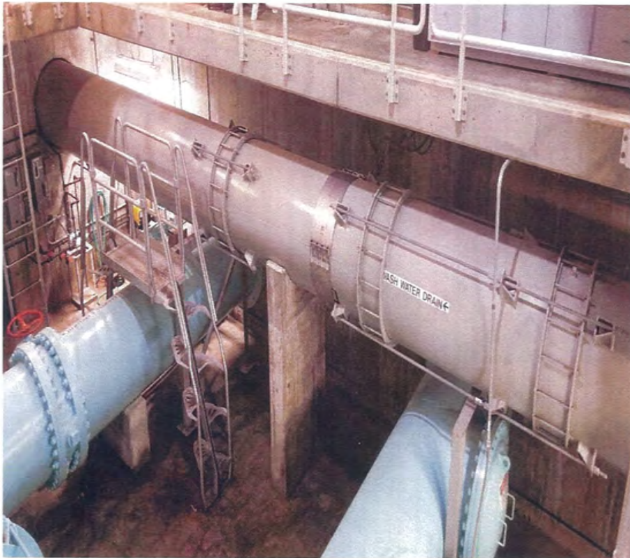
Old waste-water outfall steel concrete lined pipe
