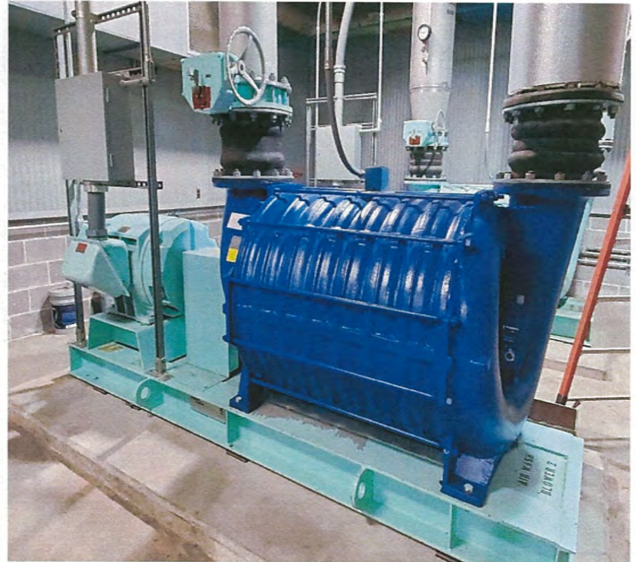
Rebuilt blower unit
