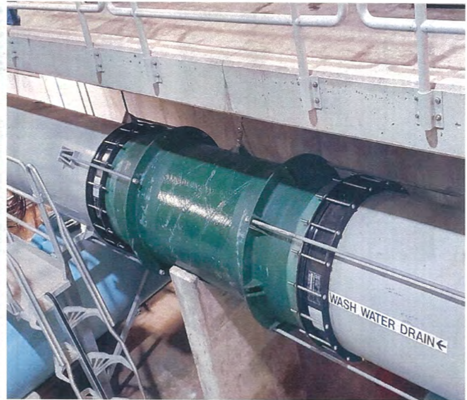
New waste-water outfall pipe fiberglass resin pipe
