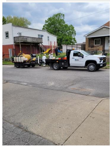
The use of pressurized water to crate a dirt slurry. The equipment can then vacuum the slurry to reveal buried utilities.
